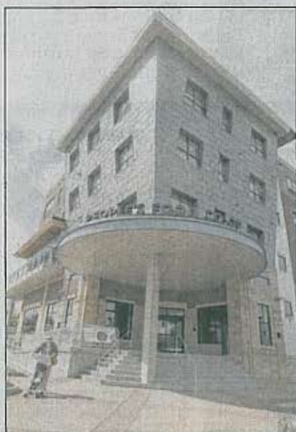
People's Food Cooperative and Metropolitan Market apartment complex building opened Tuesday at 519 First Ave. S.W.
